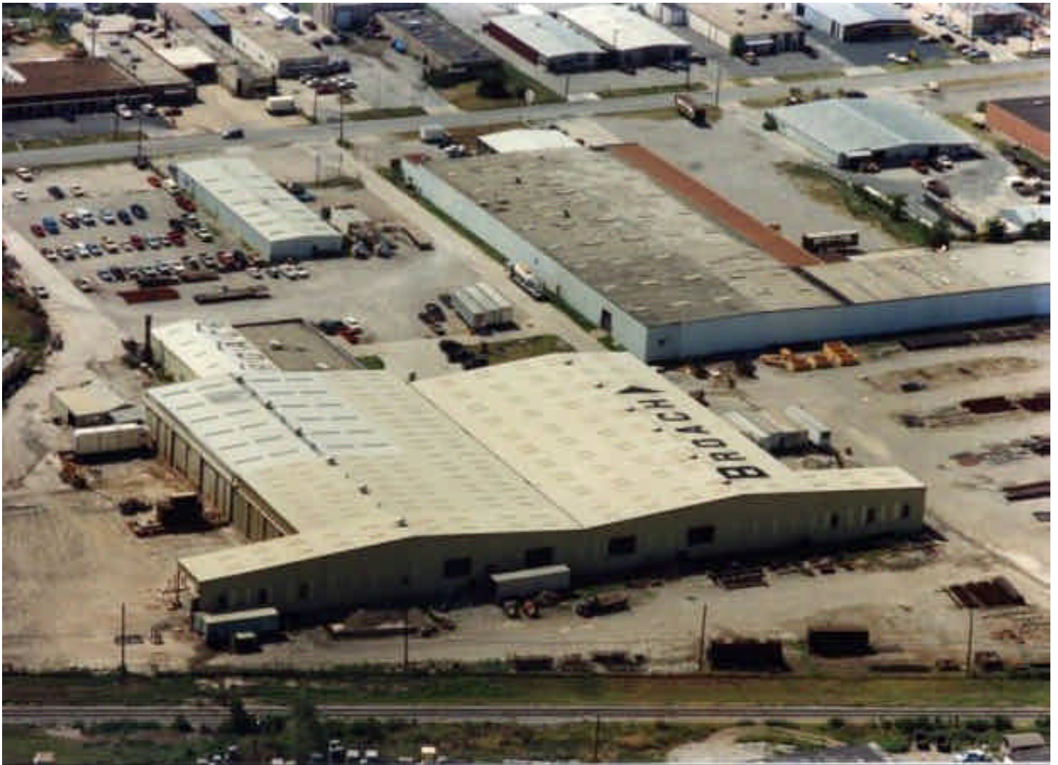
Broach Manufacturing Complex
